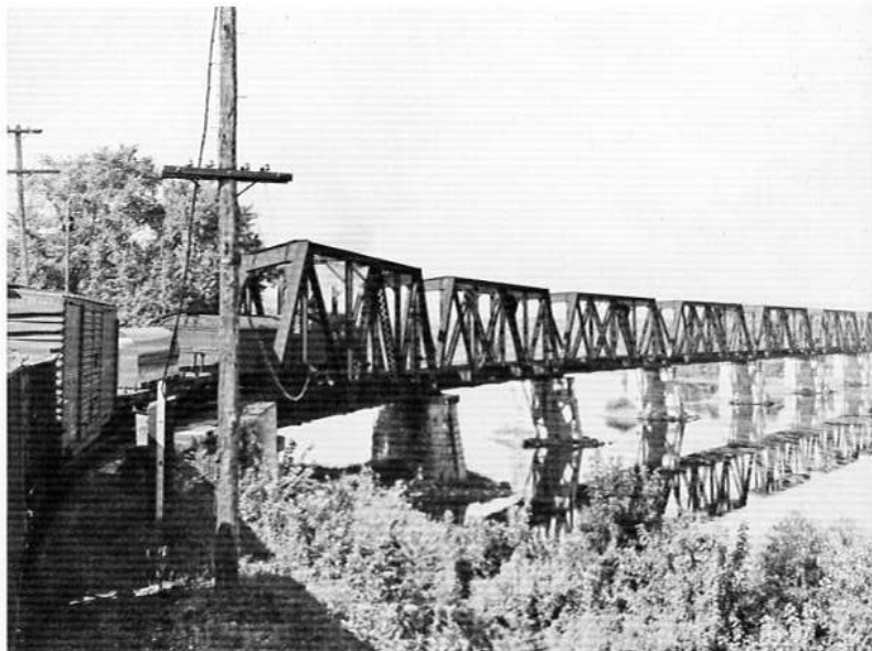
Ithaca Branch of the DL&W was connected with the mainline in Owego by a 1,000-foot, eight-span bridge over the Susquehanna River. Bridge was demolished in 1959 after DL&W mainline between Vestal and Corning was abandoned.
